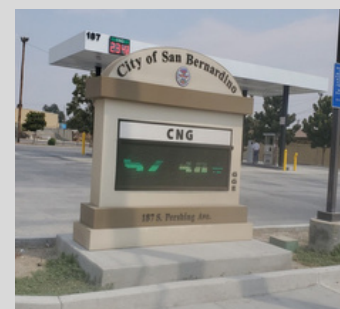
New CNG Fueling Stations
