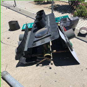
Street Light Replacement at E. Baseline St. & N. Windsor Dr.
